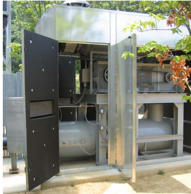
The discharge silencer pictured above is much larger than a standard discharge silencer and provides an additional means for minimizing turbulence.
